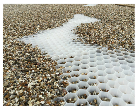
Reinforcement stabilisation grid
