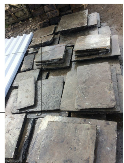
Salvaged flagstones to form new path and separator strip to front wall
