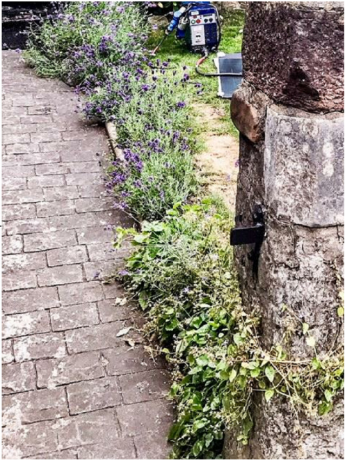
Existing concrete path with stamped paviour effect
